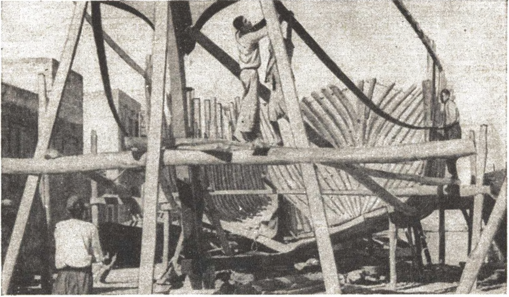
The island craft are built to-day very much in the same way as they have always been.
